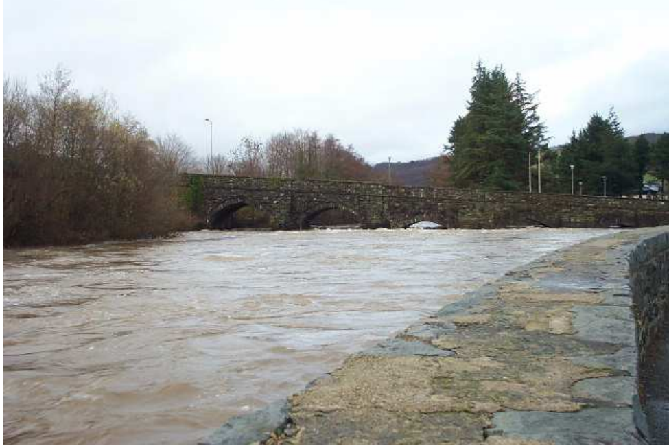
Figure 1.8: Flood defence wall alongside Bont Fawr. Flood event of 4 February 2004.
