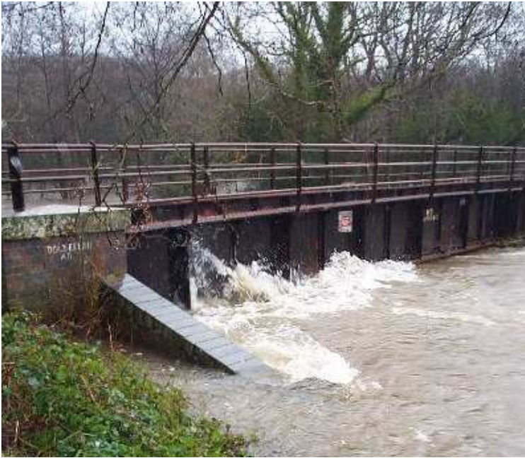
Figure 1.4: Disused railway bridge at the tidal limit of the River Wnion, Dolgellau. This is likely to be the site of the 1880 bridge failure.
