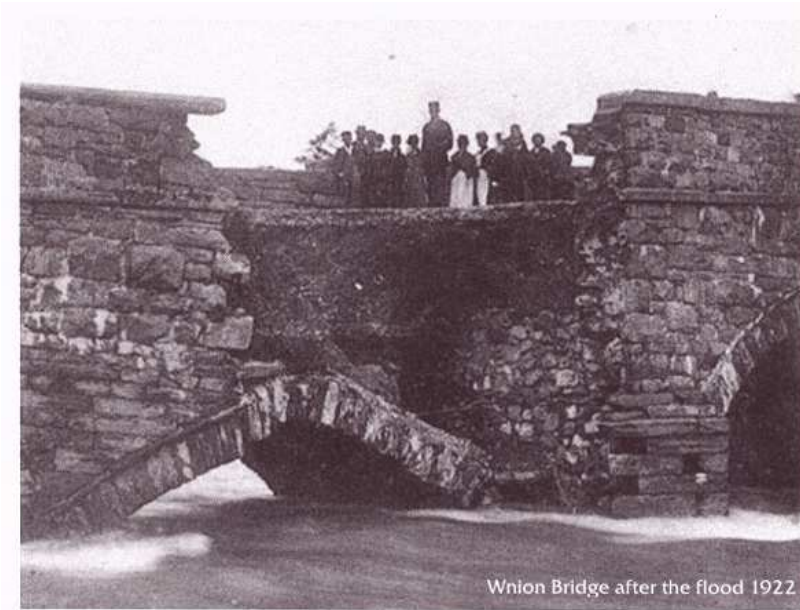
Figure 1.6: Damage to Bont Fawr, Dolgellau, September 19, 1922. (photo: Richard Morgan collection)
